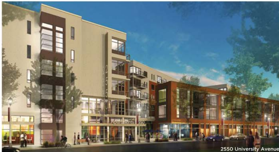
Stevens has teamed up with the Mullins Group, LLC and Eppstein Uhen Architects on this multi-family, mixed-use apartment building. It is the largest privately funded project currently under construction in the City of Madison.
